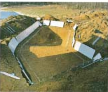
FOXGARD® components are placed in position around the pool.
