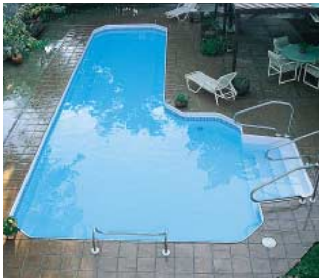
This Fox 36' x 9' Custom Lap Pool was constructed by South Plains Pool & Patio, TX
