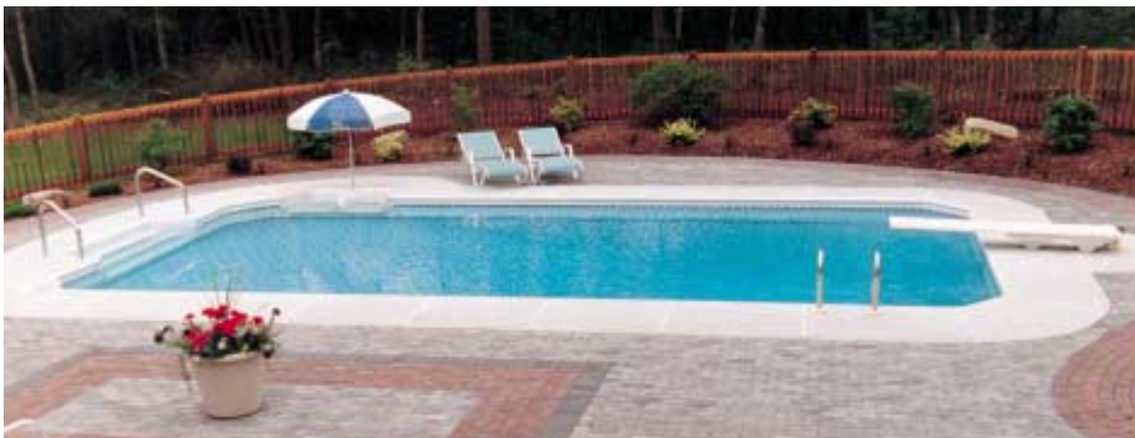
This Fox 16' x 34' Rectangle was constructed by Sparklynn Pools, Inc. NH
