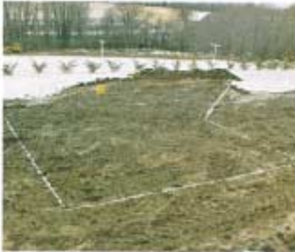
After selecting the ideal location, the pool is laid out.
