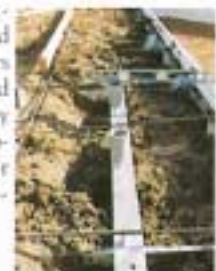
The liner is installed and the pool is ready to be filled. In this case, the pool could be completely filled before backfilling or pouring the deck, further evidence of the Fox statement that the pool is self-supporting.
