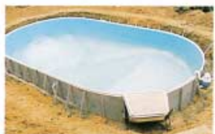
The liner is installed and the pool is ready to be filled. In this case, the pool could be completely filled before backfilling or pouring the deck, further evidence of the Fox statement that the pool is self-supporting.
