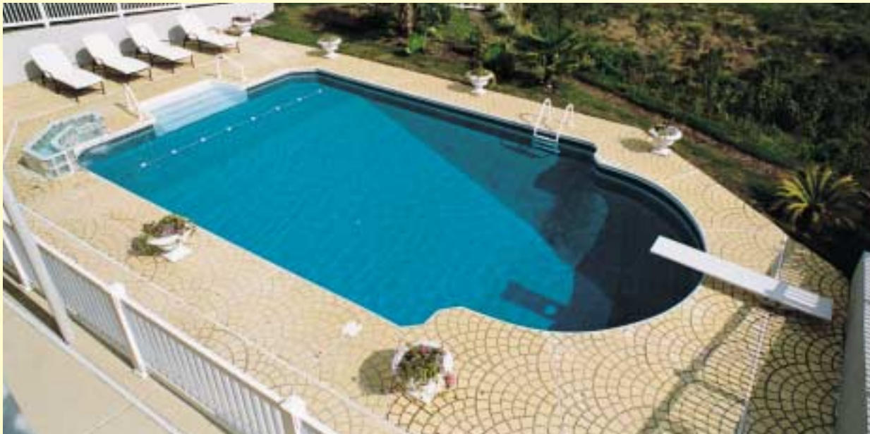
Baxter Construction Company of Virginia Beach, Virginia Beach, VA built this 20' x 36' Ionic with stairs, ladder and Fox all-white rails.
