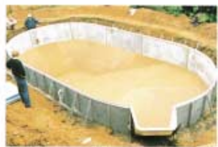
The Fox recommended construction method applies to rectangular and free form pools. Here a sand, vermiculite or sand/cement bottom is shaped and smoothed to the dimensions provided on the Fox "dig" drawing.
