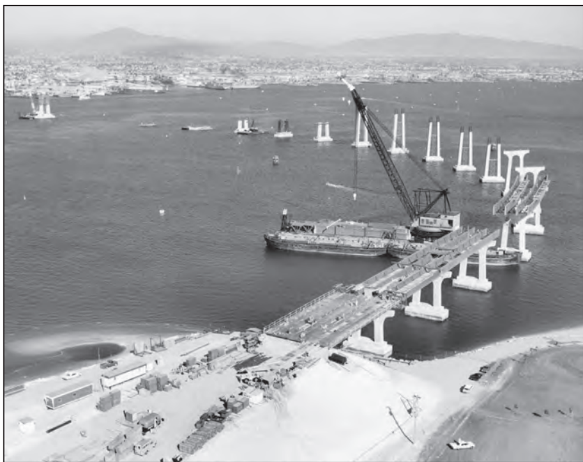
Construction of the Coronado Bridge, circa 1969
