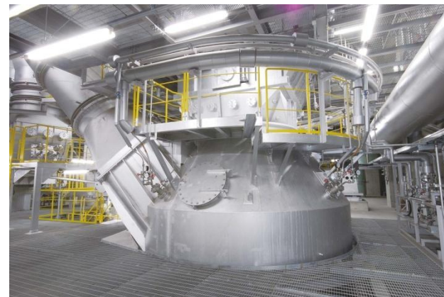
(Direct Melting System / Gasifier)
