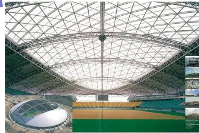
Building Construction & Steel Structures
