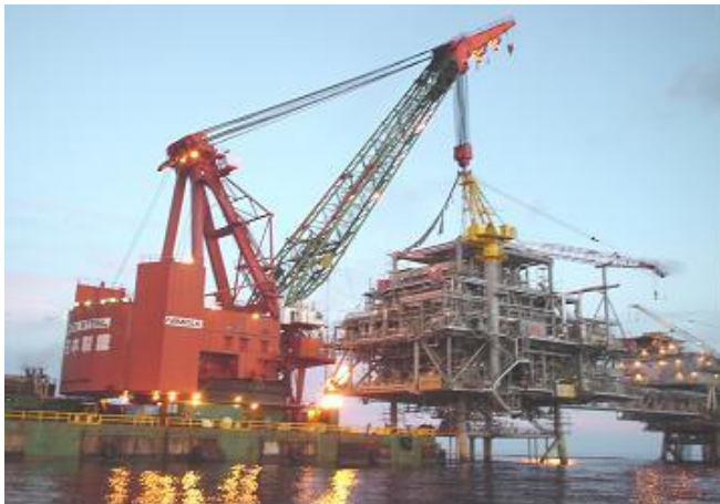
Energy facilities, Civil Engineering & Marine Construction
