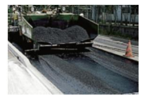
Asphalt paving
