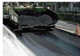
Asphalt paving
