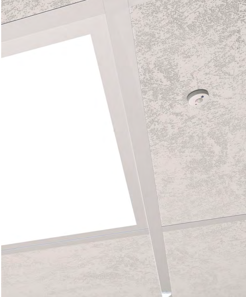
Below the Ceiling
