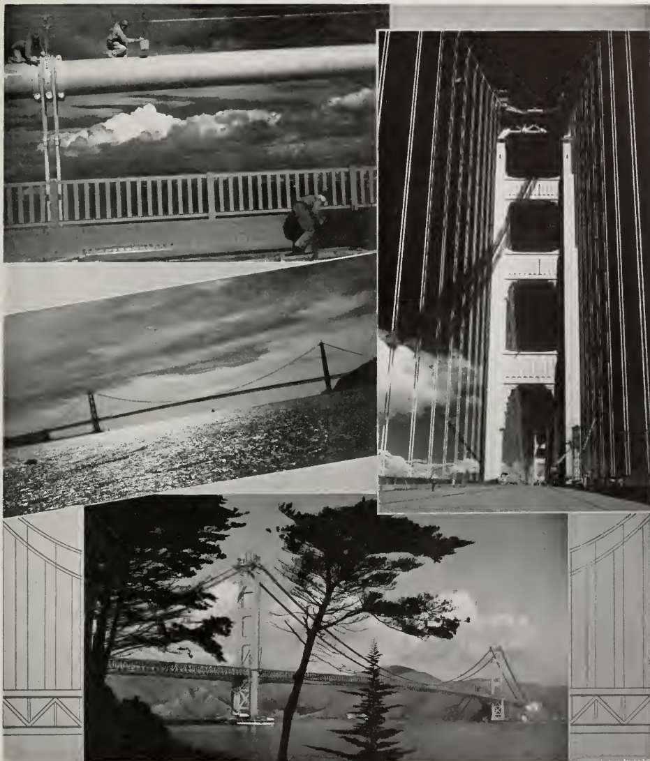
Beauty of the Golden Gate Bridge is exemplified in these artistic photographs. Upper left, cloud effects and cable workmen. Left center, looking out the Golden Gate in the moonlight. Upper right, an idea of the massiveness of the South tower by night. Lower, an artistic view from the San Francisco shore.
