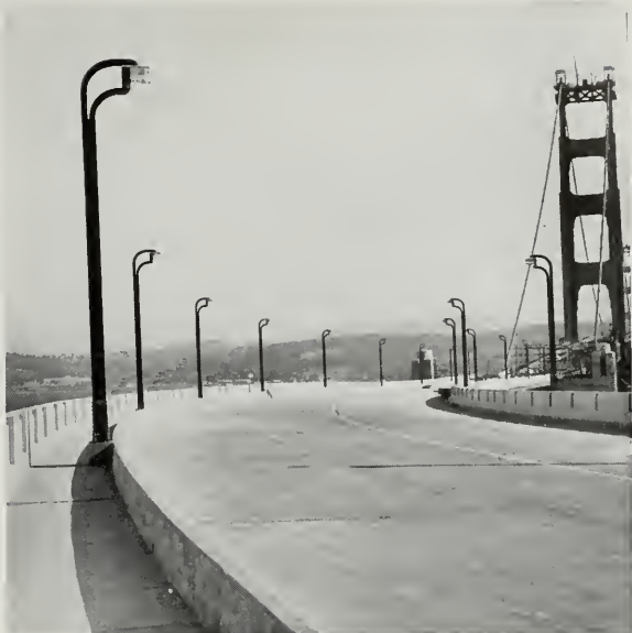
MARIN APPROACH TO BRIDGE
