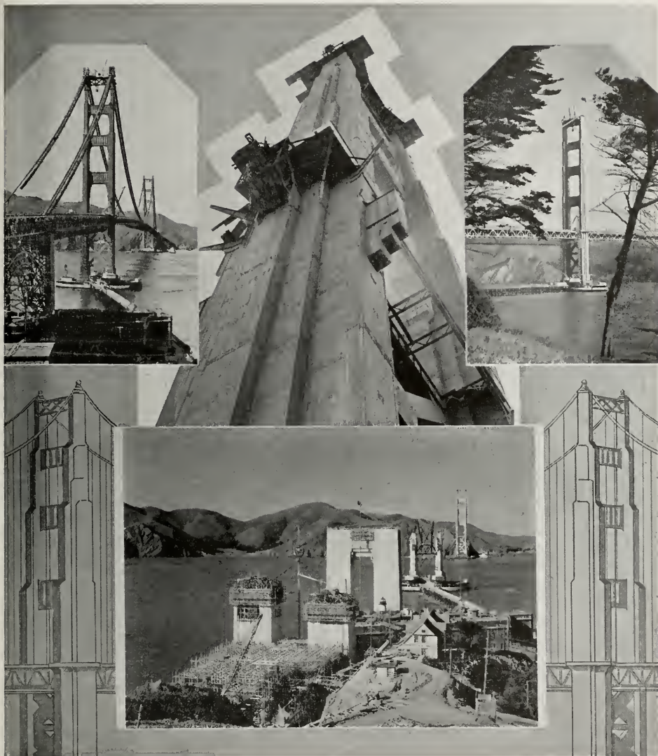
Upper left—Bridge from above Old Fort Winfield Scott. Upper center—Massiveness of the giant towers. Upper right—San Francisco tower. Below—General view, showing San Francisco anchorage during course of construction, in the foreground, with the South pylons, start of work on South tower, and Marin tower in distance.
