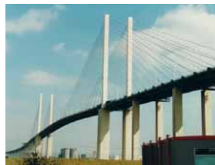
Figure 12.9: Cable stayed bridge
