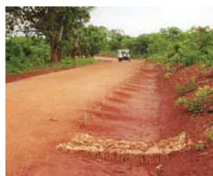
Figure 11.5: Scour check constructed from wooden stakes with a masonry apron
