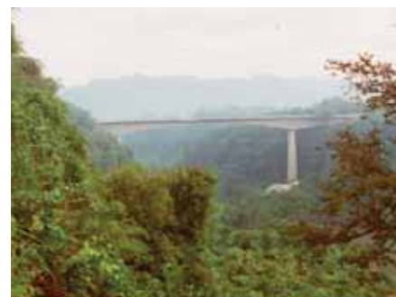
Figure 12.8: Concrete box girder bridge
