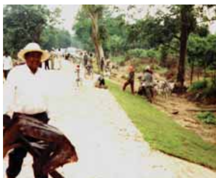
Figure 11.6: Turf is being placed on this embankment to prevent erosion
