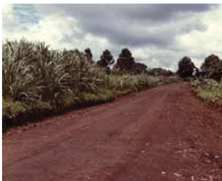
Figure 9.2: Well shaped earth road
