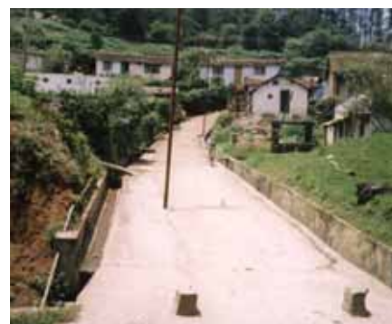
Figure 11.4: The short and steep access road has been constructed with concrete drains to prevent erosion
