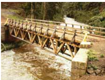
Figure 12.6: Modular timber bridge
