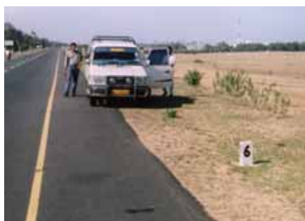
Figure 11.2: Sealed shoulders together with low embankment slopes ensure that the pavement remains dry and strong.
