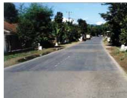
Figure 8.5: Rumble areas on entry to village, Indonesia
