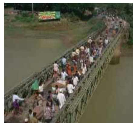
Figure 12.4: Congestion on single lane bridge
