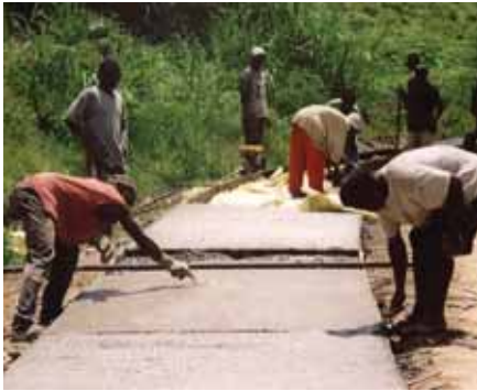
Figure 7.2: Labour-based road works, Tanzania
