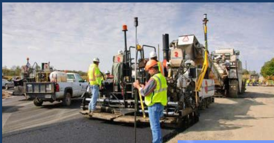
Stringless HMA Paving
