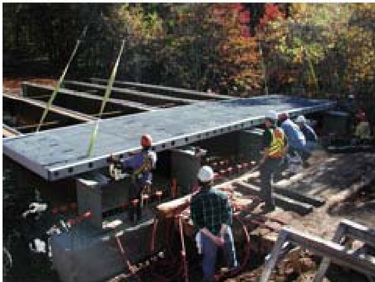
Composite bridge decks ( www.cobrae.org )
