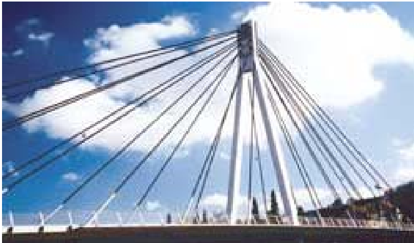
Bridge cable stays ( www.compositesworld.com/ct/issues/2006/February/1180 )
