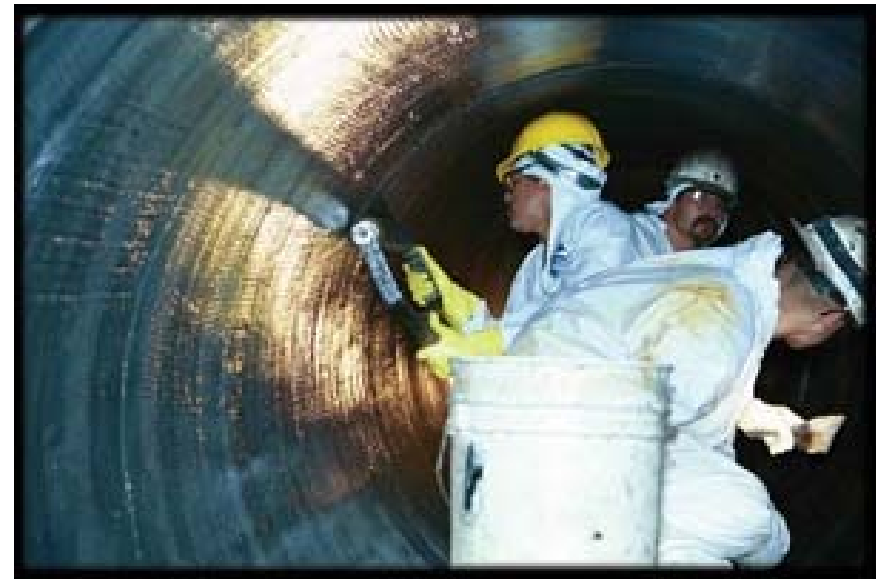
Lining large dia piping ( www.fibrwrapconstruction.com )
