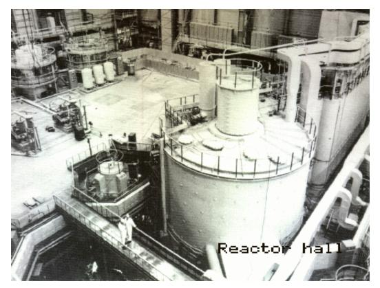
BN-350 was designed for the dual purpose of producing electricity (150 MW) and desalting water (120,000 m<sup>3</sup> fresh water/day), which corresponds to a total power generation of 350 MW(electric).
