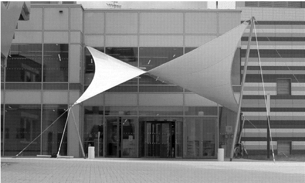
Fig.1: A tensegrity shelter built at Brno University of Technology, Brno
