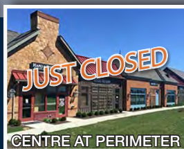
CENTRE AT PERIMETER DUBLIN, OH CONFIDENTIAL
