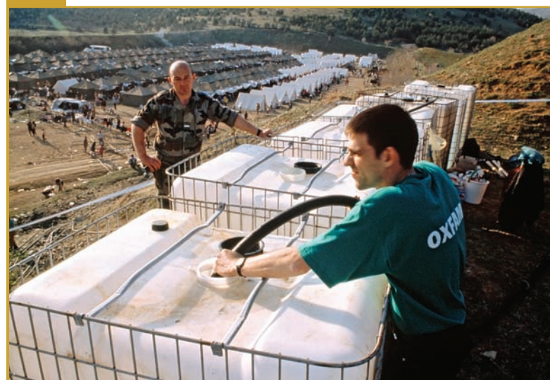
The British aid agency, OXFAM, installing a water supply system at Stankovac 1 near Brazde. Stankovac 1 is the first major reception site established by NATO, with UNHCR's support, several kilometers from the Kosovo border. (UN Photo #76370 by JJ Davies, April 2009)
