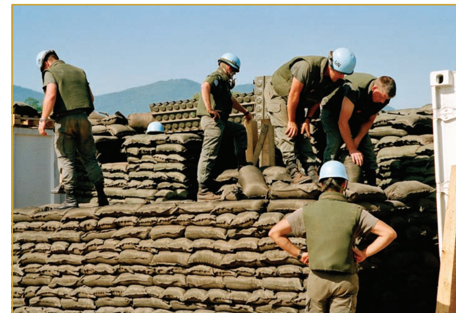
French soldiers building a sandbag bunker at Sarajevo Airport. (UN Photo #121850 by John Isaac, September 1992)
