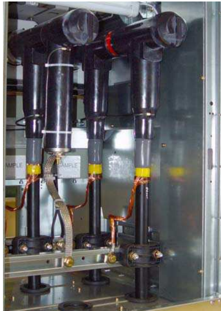
Fig. 99: Mounted surge arrester (example)
