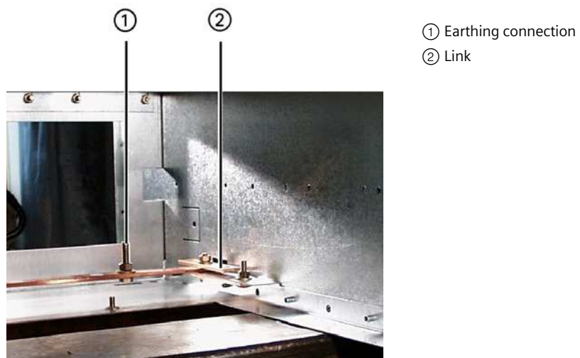
Fig. 78: Earth connections
