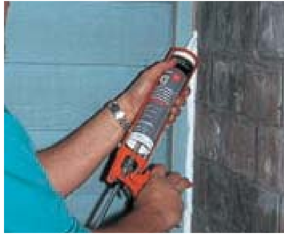
Caulk upward, pushing a bead of paintable caulk in front of the nozzle as you work.
