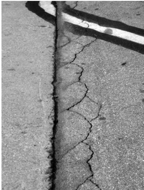
◀ Joint sealant needs replacement at several locations. Follow with new surface treatment on apron.
