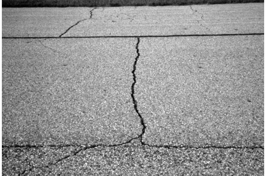
▶ Right angle cracking forms blocks.
