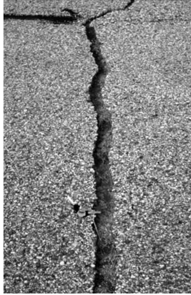
▲ Wide cracks with no sealant.
