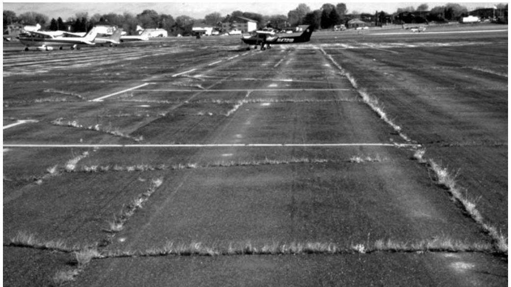
▶ Right angle cracking forms blocks.
