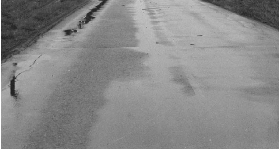
▲ Even slight rutting is evident after a rain.
