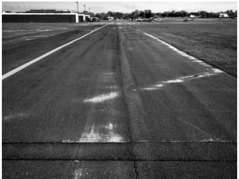
▼ Worn sealcoat needs new surface treatment.
