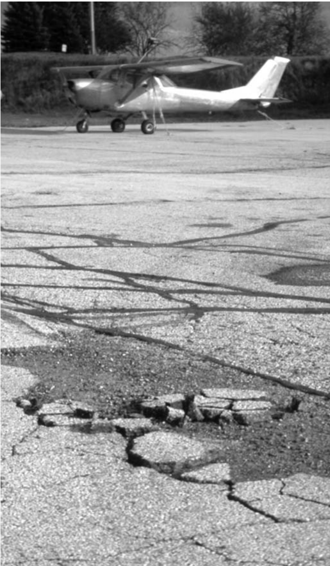
Complete pavement failure. ▼
