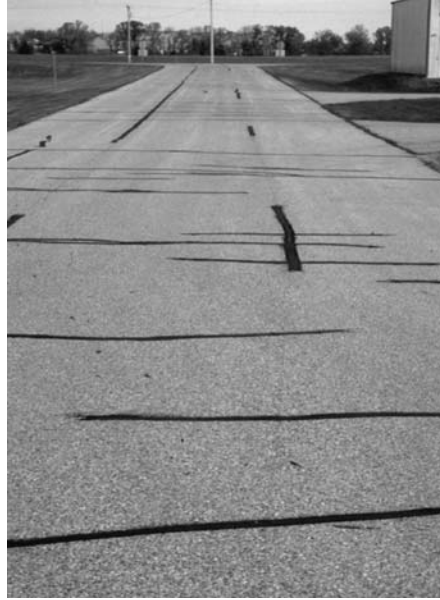
▲ Widely spaced, well-sealed cracks.
