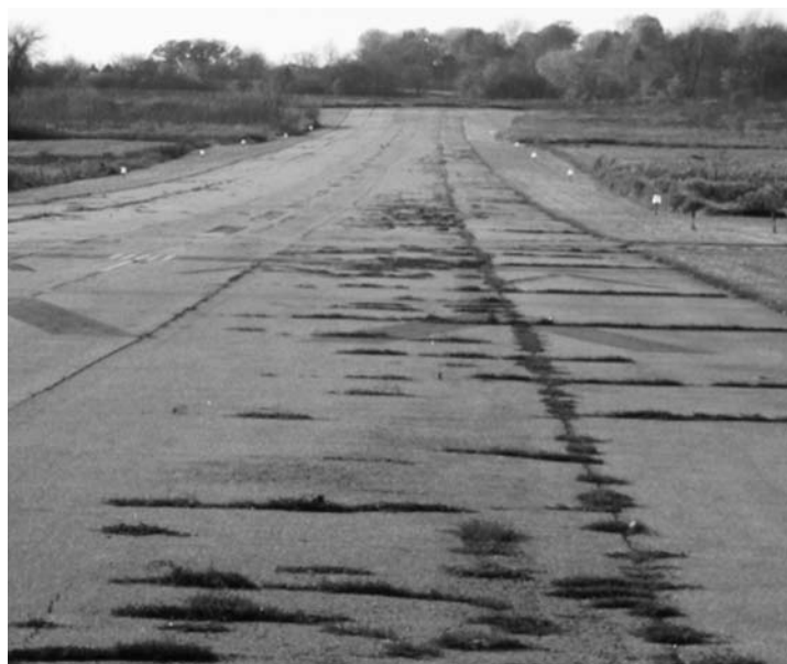
▲ Severe cracking and deterioration.
