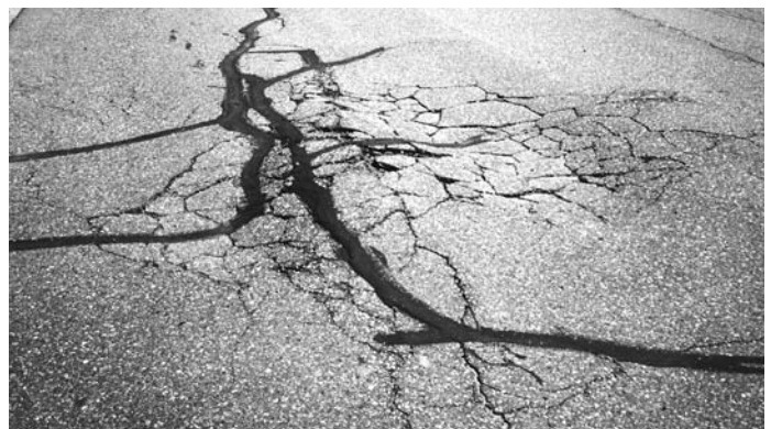
▲ Frost heave damage from spring break-up.
