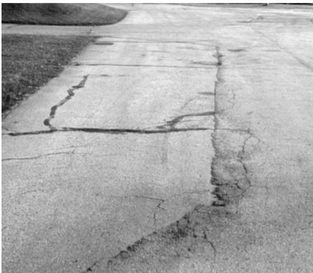
▼ Overlay repair with edge raveling and cracks.
