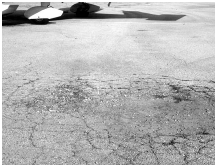
Complete pavement failure. ▼
