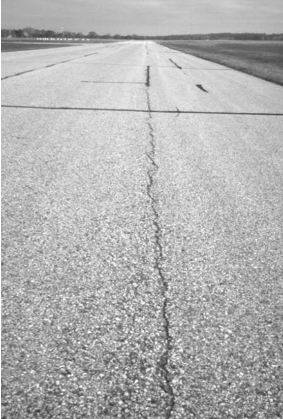
◀ Moderate raveling. Joint needs sealing.
