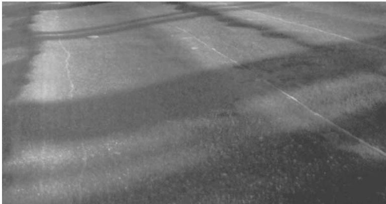
▲ Even slight rutting is evident after a rain.
