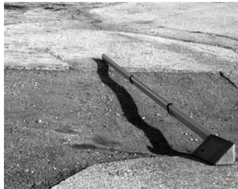
▲ Frost heave damage from spring break-up.
