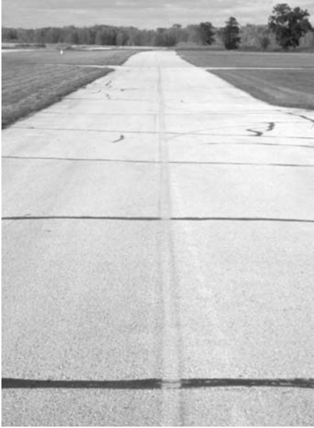
▲ Widely spaced, well-sealed cracks.
