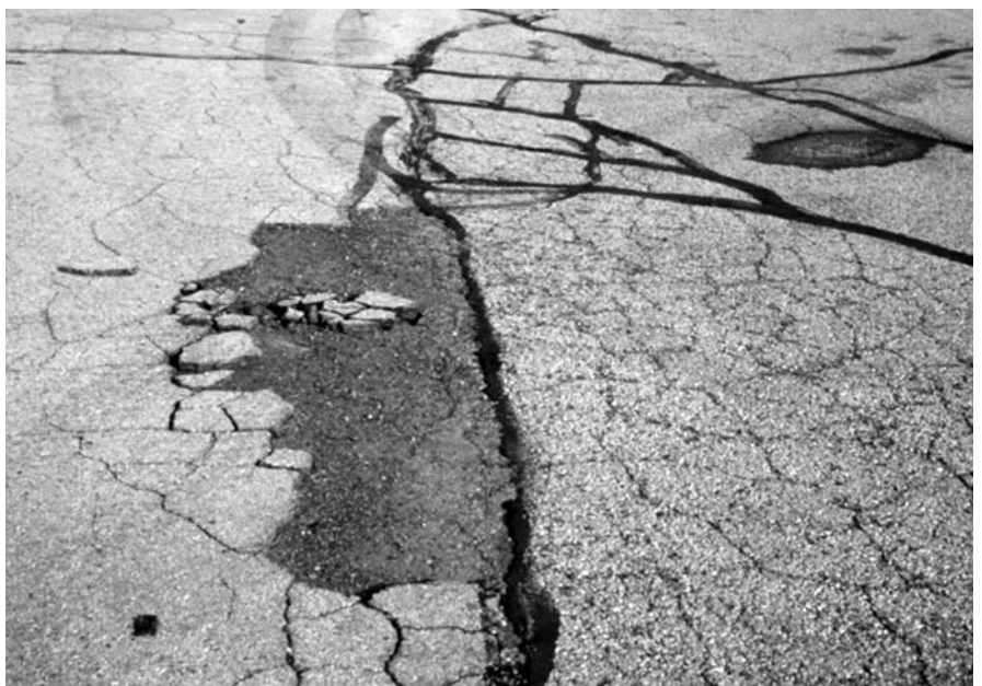
▶ Extensive failed pavement and debris.
