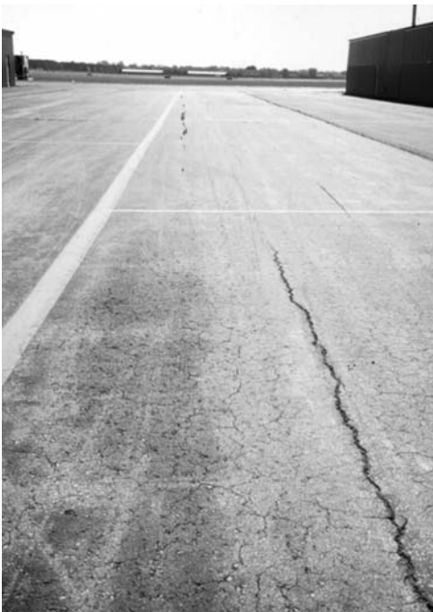
▶ Severe cracking and edge distress.
