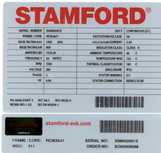
FIGURE 1. GLOBAL STAMFORD AC GENERATOR NAMEPLATE, COMPRISING RATING PLATE AND TRACKING LABEL
