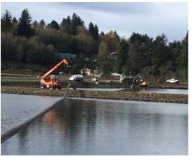
Photo: The HDPE pipeline shown lofted during pullback
