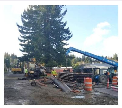
Photo: The HDD Rig and Entry Pit shown working around the Coast Redwood. In this photo, the conductor casing and 18-inch product pipe can be seen.
