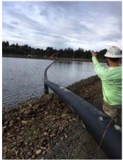
Photo: Pullback of the 18-inch pipe across the lagoon
