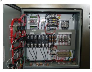
WARNING Do not turn on main power to the chiller system until all of the electrical connections are confirmed to be tight.
