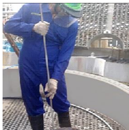
Fig. 4. Hydro-jet cleaning of tubes in progress.
