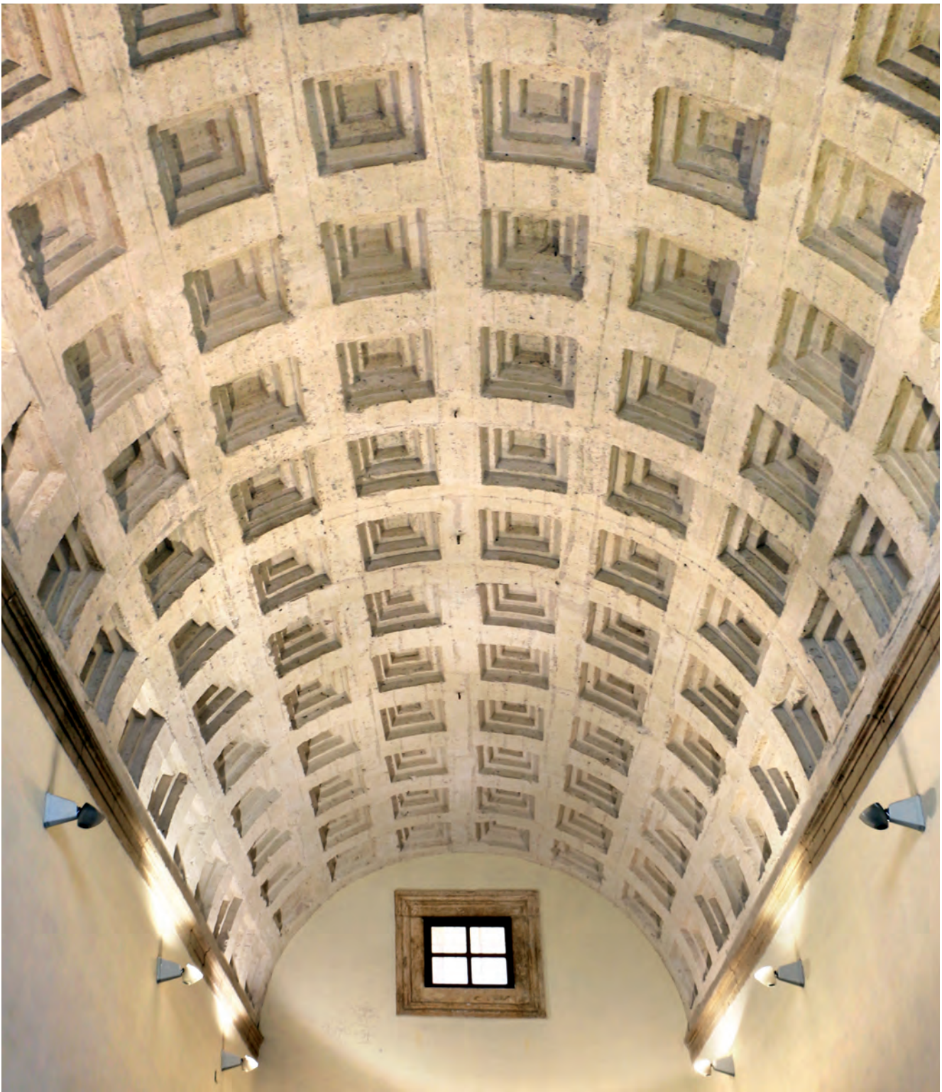
Fig. 1. Francesco del Borgo, Coffered barrel vault of the vestibule of the Palazzo Venezia , Rome, c.1466 (Photo: Sailko, Wikipedia Commons).
