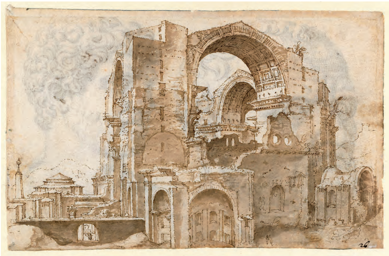
Fig. 3. Maerten van Heemskerck, View of Saint Peter's in construction with Bramante's large concrete vaults connecting the crossing piers , c. 1532-36, Kupferstichkabinett, Staatliche Museen zu Berlin, Berlin, Heemskerck-Album, vol. I, fol. 13r (Photo © Kupferstichkabinett, Staatliche Museen zu Berlin, Berlin).
