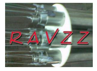
Video -New copper leads being connected by shortening the length of previous leads
