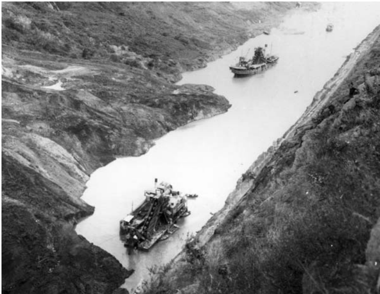
Dredges work at the Cucaracha slide in December 1913 after the flooding of Culebra Cut three months earlier. Though less glamorous than the steam shovels, these waterborne machines made their own large contribution to moving dirt for the canal.
