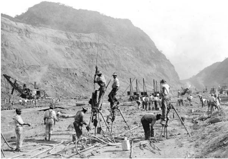
Workers operate tripod drills in the foreground. Other crews filled the holes with dynamite. The resulting explosions loosened the earth for the steam shovels, visible at work in the background.
