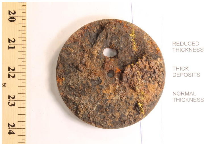
Figure 5: Photograph showing the hole in the tank bottom as viewed from the outside of the tank. Note-circular hole in center is a drilled hole.
