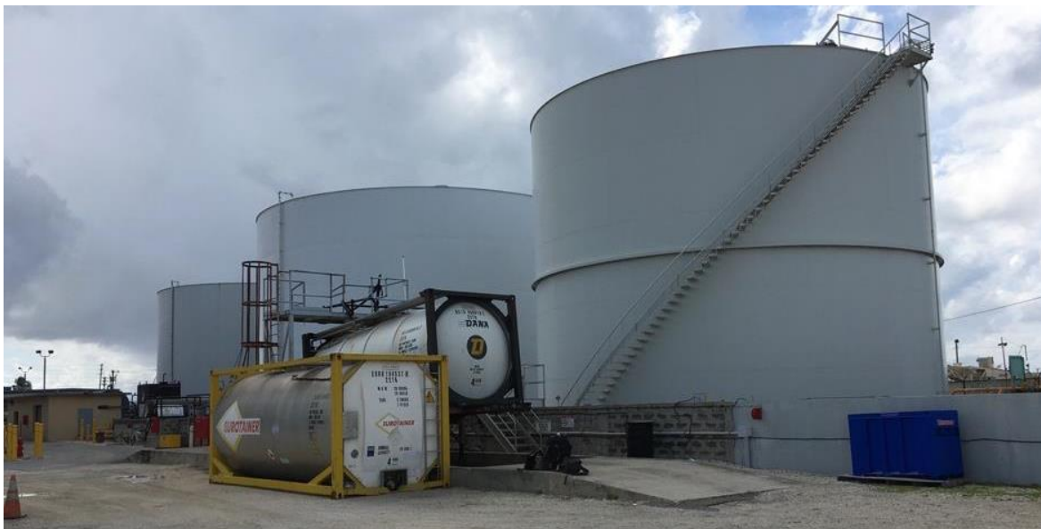
Figure 2: Photograph showing Fuel storage tanks.
