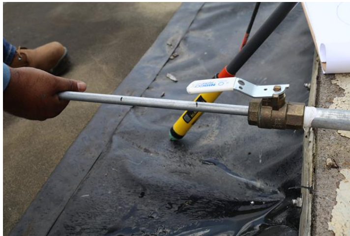
Figure 18: Photograph showing placing of auxiliary electrode in between the tank bottoms.
