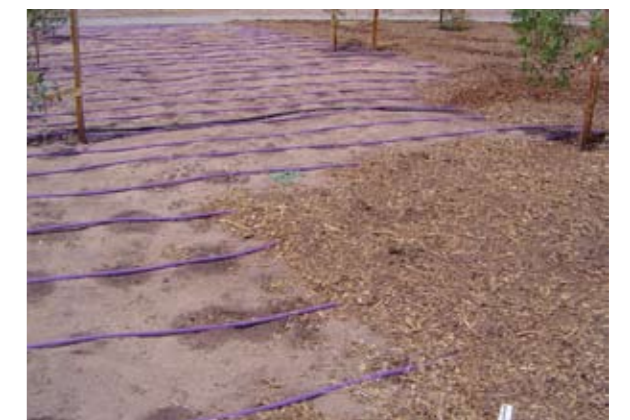
Recycled Water Irrigation
