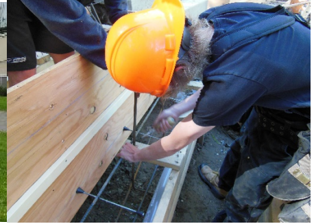
Carpentry at OC (June 2017)
