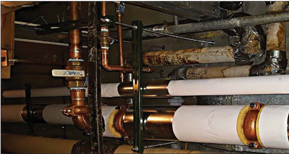
New vertical riser and valves, with old lines in the background.
