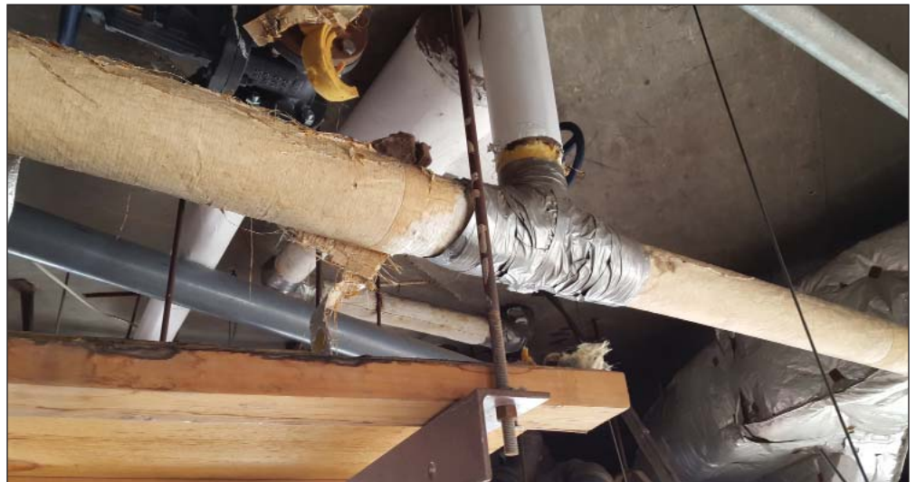
A typical vertical riser prior to replacement project.
