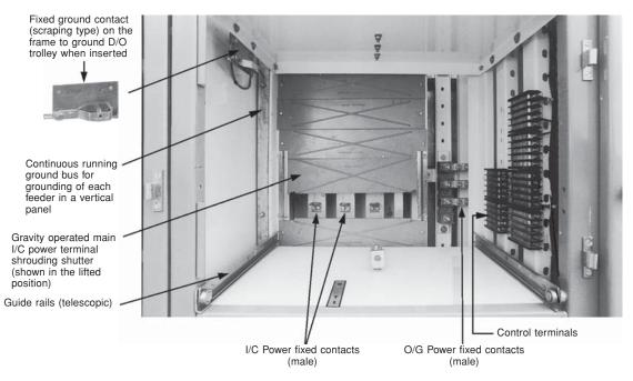
Figure 13.35 View of a module of a fully drawn-out MCC showing grounding arrangement through a continuous running ground bus
