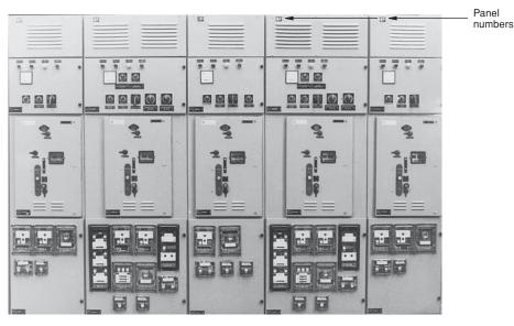
Figure 13.9(a) A typical cubicle-type power control centre (Courtesy: ECS) (now Havells India)
