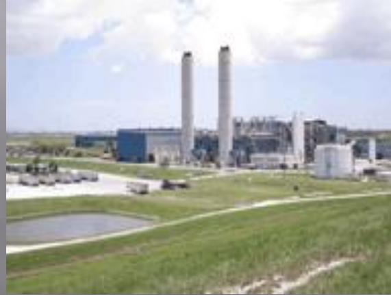
EFW Energy From Waste
