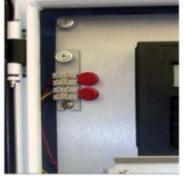
Figure 58. Metal Oxide Varistors
