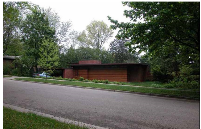
Figure 11b View from the street side - site is sloping towards the east side
