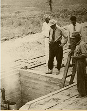
Figure 7: Wright watches the testing of the floor heating system source: Usonia 1 Jacobs House web, http://www.usonia1.com/01_hist.html
