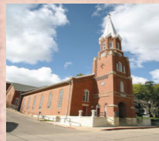
ST. MARY PARISH 400 Franklin St. Galena, IL
