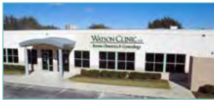
Bartow Building B
