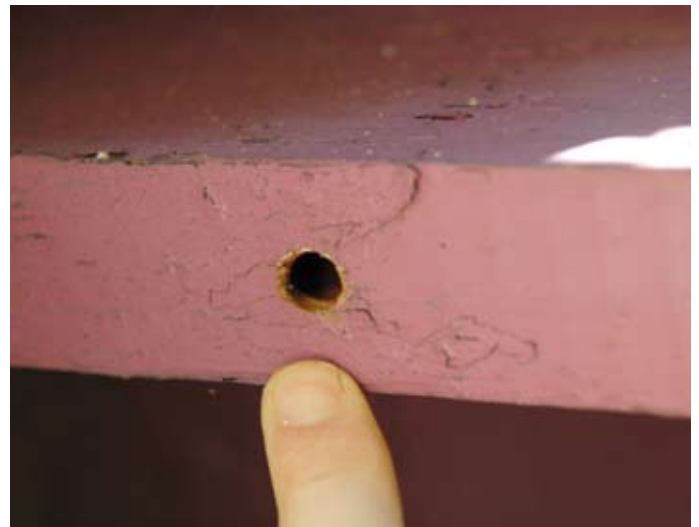
A carpenter bee hole in a rafter. Carpenter bees are a common pest of log homes.
