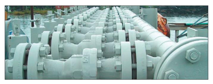
PBV® Flanged Floating Ball Valves installed in a typical manifold application.
