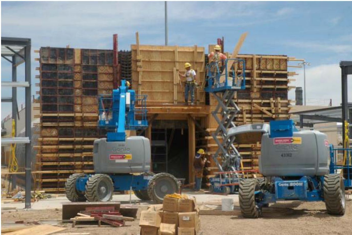
Workers install formwork on one of the Munitions Service Magazines.
