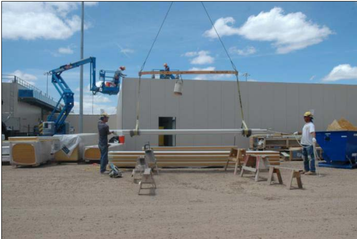
Workers install roof panels atop the Energetic Service Magazine corridor.
