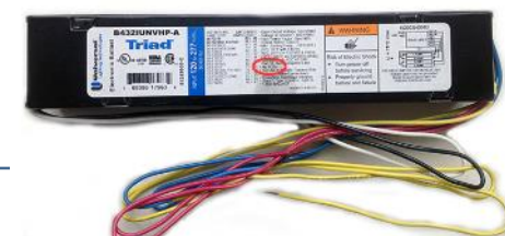
A typical Non-PCB containing fluorescent light ballast. The ballast has a "No PCBs" marking on the top of the ballast and the text "electronic ballast". Only magnetic fluorescent light ballasts contained PCBs.
