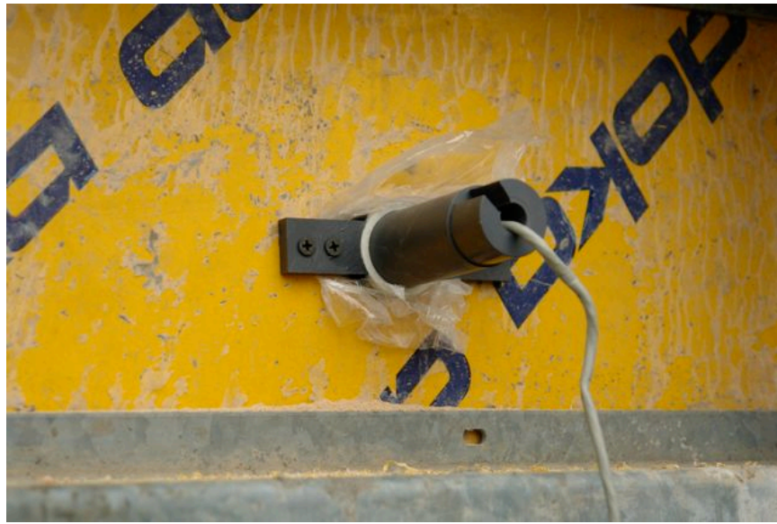
Figure 3 —Bracket with Pressure Transducer Attached to Formwork
