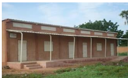
A completed two classroom block.
