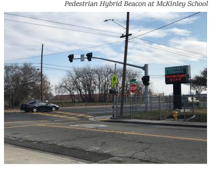
4C.05 [Warrant 4, Pedestrian Volume] and/or 4C.06 [Warrant 5, School Crossing], but a decision is made not to install a traffic control signal." PHBs should be installed at an intersection, or at the junction of a roadway with a driveway, or at least 100 feet from side streets or driveways that are controlled by STOP or YIELD signs.
