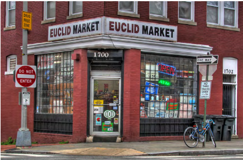
14. Exterior photograph of the Euclid Market building in Washington, D.C. taken on April 6, 2008 before demolition. Photo by Ron Roberson.
