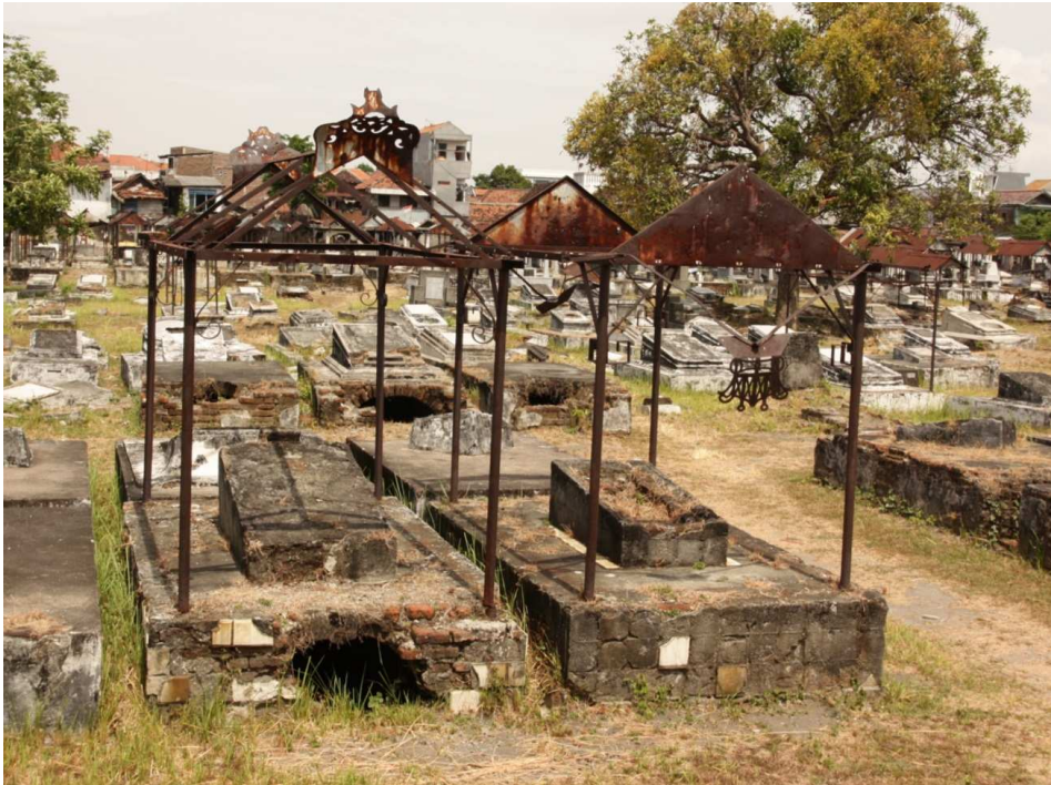
Two type 3 monuments, roofed, no fencing and in a poor condition. Can be valued as 1 (depending the persons buried here)
