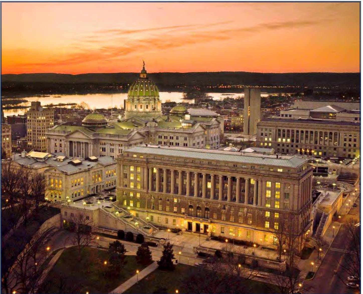
Pennsylvania Capitol Complex looking North. Site of three ongoing GESA projects to reduce energy consumption.
