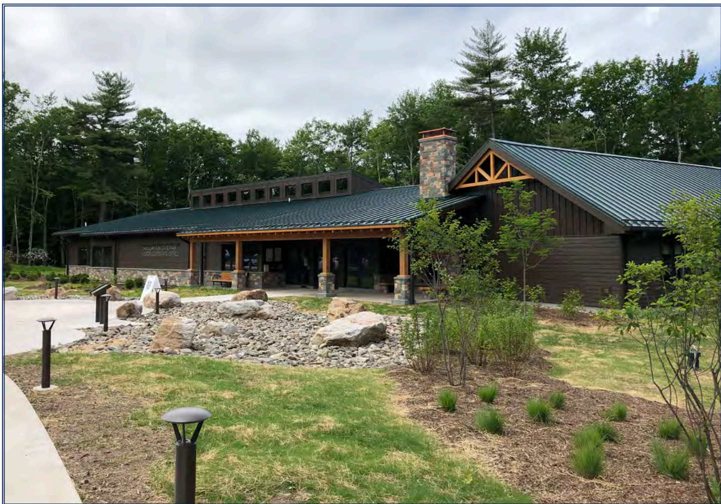
Hickory Run State Park Visitor Center and Office. LEED green building certification anticipated in 2021.
