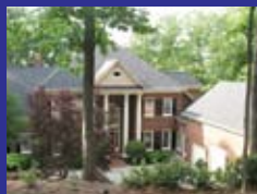
Cramer Mtn! Executive home! 3 levels! 6 BR! Beautiful views! Every Detail! Separate Apartment! $375,000
