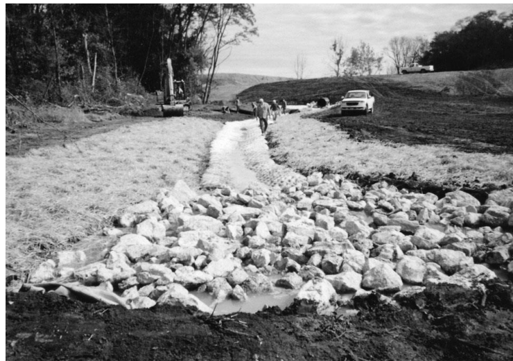
Photo 8. Downstream Terminus of the RECP Lining During Construction, looking northeast
