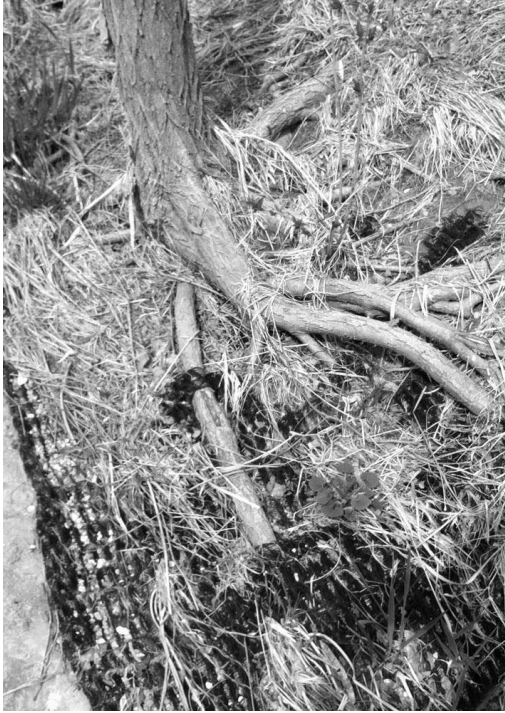
Photo 3. Tree Roots Anchoring HPTRM
