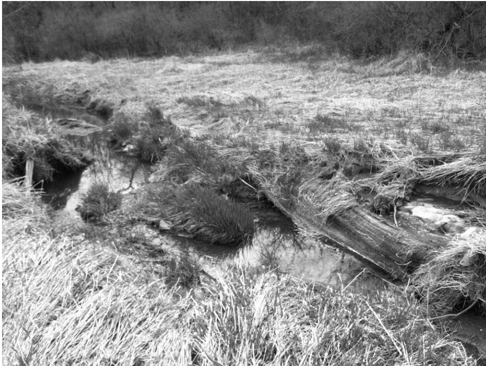
Photo 9. Near Downstream Terminus of RECP Lining, looking southwest
