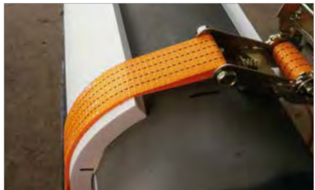
Crushable Foam Wrap panels shown during installation.
