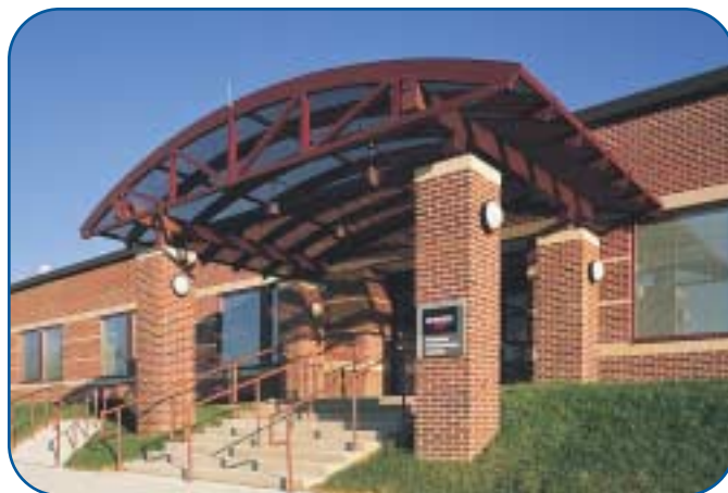
USA Technical Center, King of Prussia, Pennsylvania
