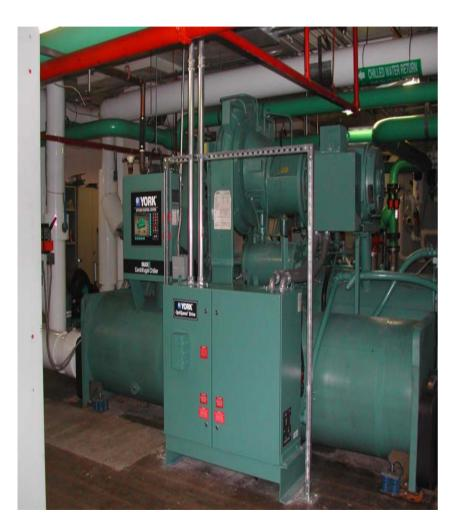
New variable speed drive chillers installed at City Hall and Mountain Creek Library to eliminate ozone depleting refrigerants and provide high efficiency chilled water.
