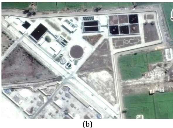
Fig.1 Ghazl El-Mahalla WWTP in (a) a general layout showing the current status and the proposed upgrading, (b) an aerial photo adapted from Google Earth, March 2018
