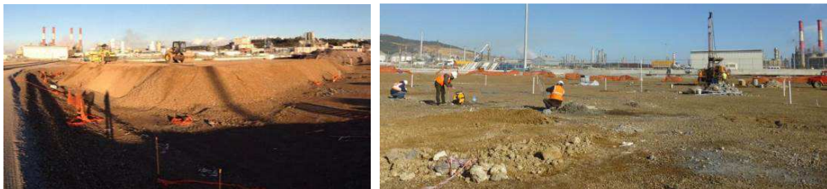
Figure 5. Test embankment and installation of instruments
