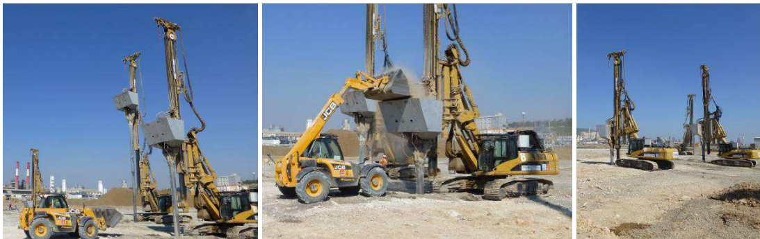
Figure 3. The construction of Impact ® RAPs.
