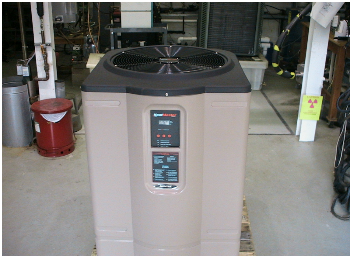
Figure 21 Hayward Model: Heat Master HML-125T electric heat pump
