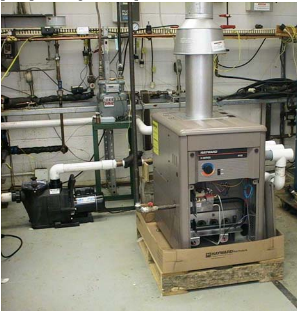
Figure 11 Baseline gas-fired pool heater in the BNL test facility
