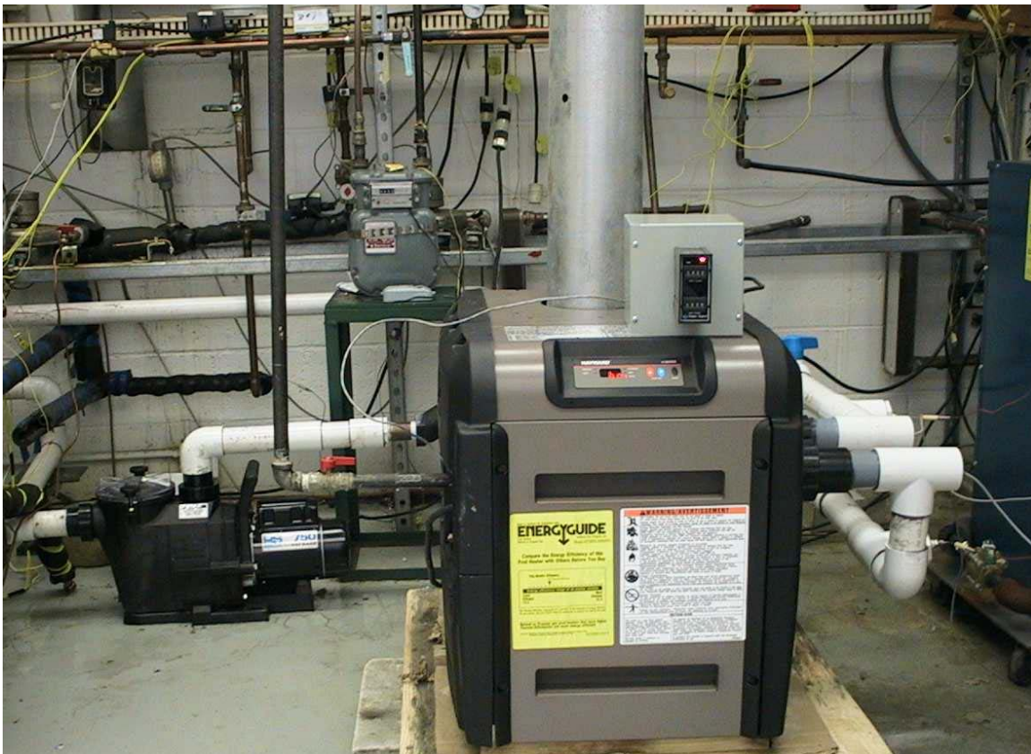
Figure 18 Hayward H150FD low NO x natural gas-fired pool heater
